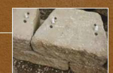
Starting with straight areas first, begin placing the second course. Center each Keystone Verazzo Stone unit over the pins on the joints of the course below in a running bond pattern as shown. Now proceed to the next layer, backfilling as you go. For drainage between units and behind the wall, clean gravel or crushed stone is recommended.
