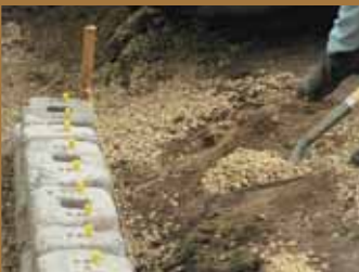
4. INSTALL FILL & COMPACTION
