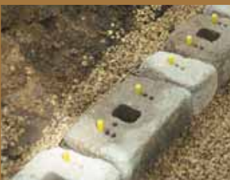
3. INSERT THE FIBERGLASS PINS
