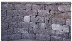
UNIT ABOVE VERTICAL UNIT SPANS TO BEAR ON EACH SIDE
